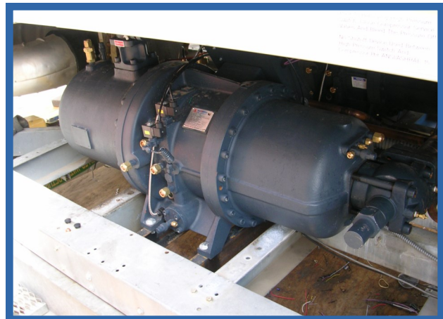
McQuay chillers upgraded with Hanbell screws and MCS Controls
