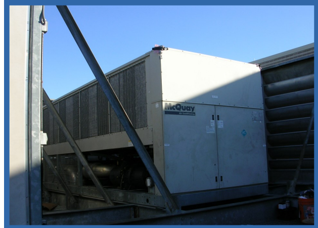
McQuay chillers upgraded with Hanbell screws and MCS Controls
